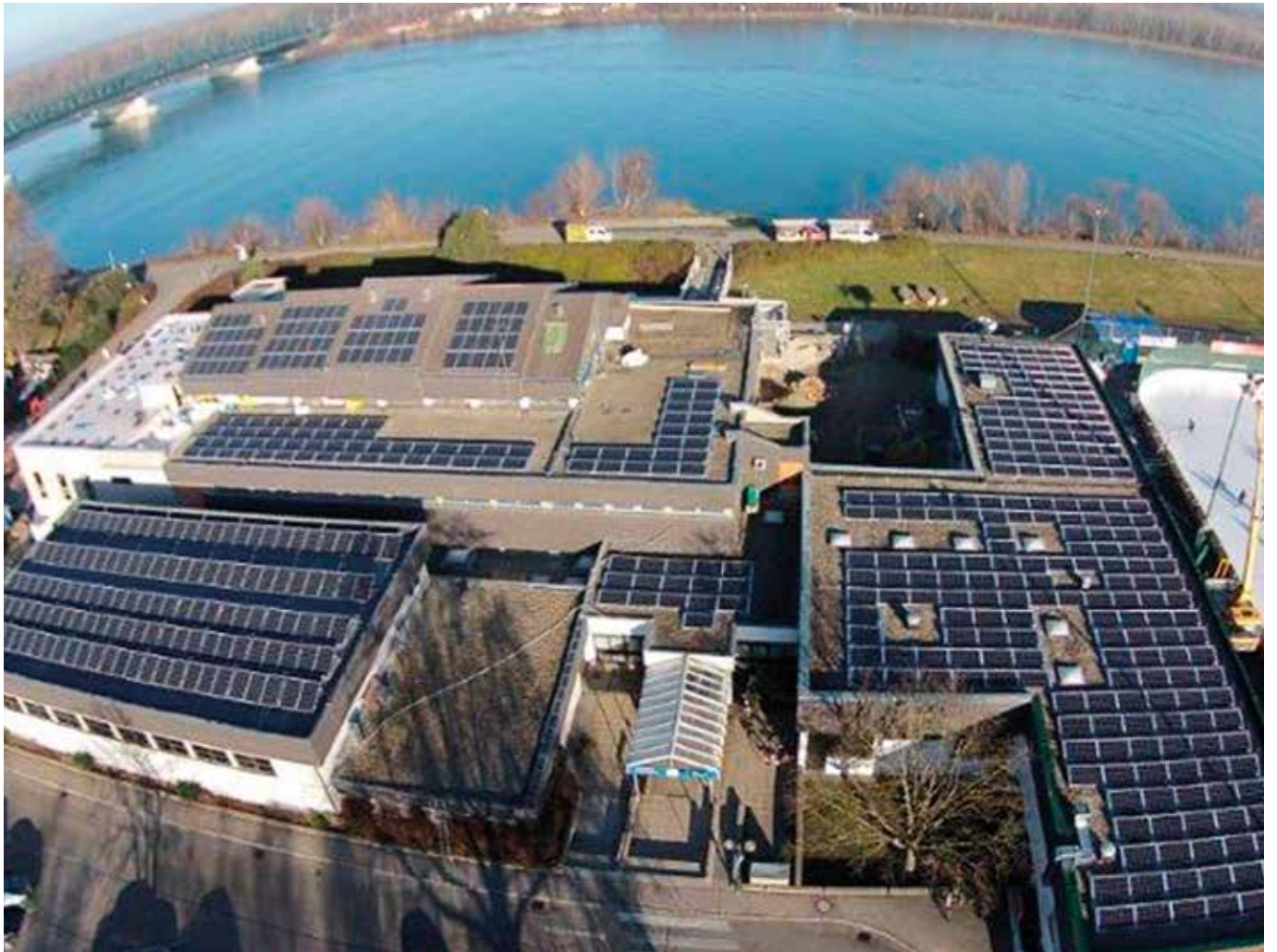
The photovoltaic system on the roof of the indoor swimming pool in Tulln, Austria can supply more than 30 households with energy.
