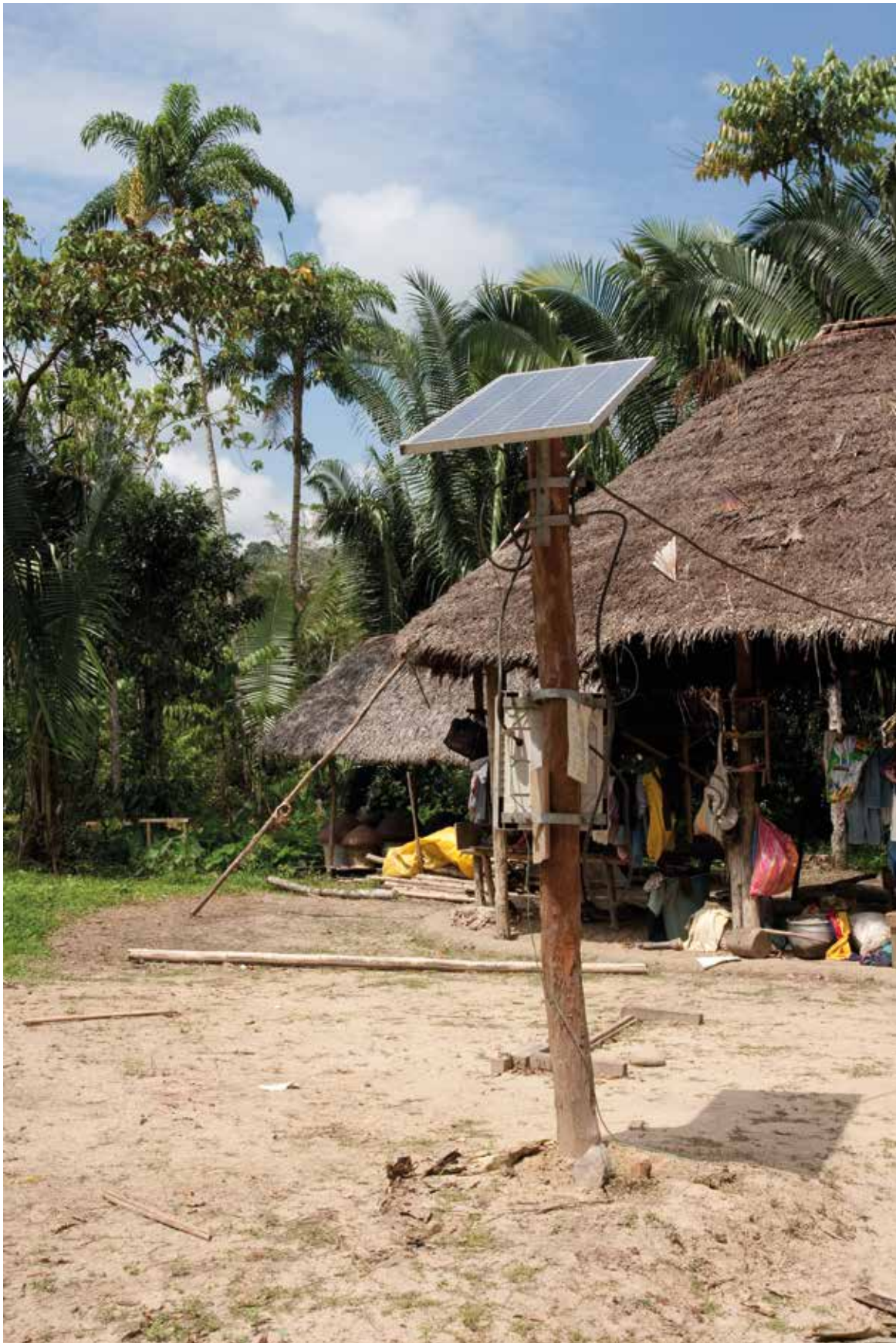
Solar panel in the Kichwa community of Sarayaku, Ecuador
