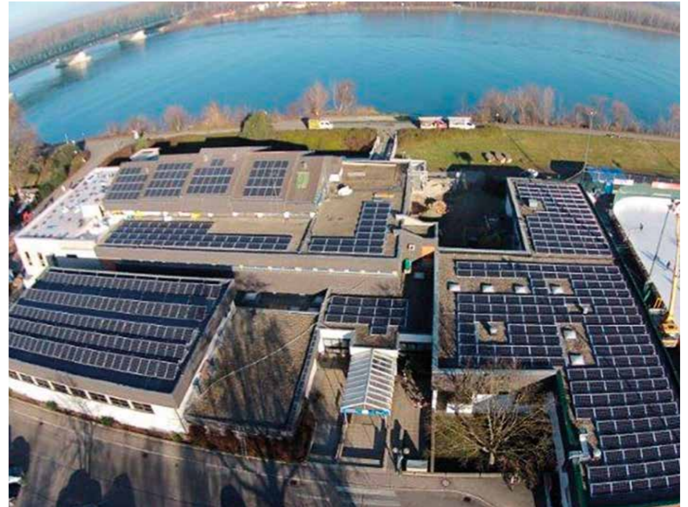
The photovoltaic system on the roof of the indoor swimming pool in Tulln, Austria can supply more than 30 households with energy.
